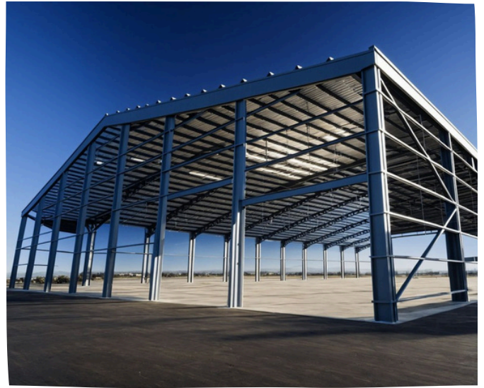
STEEL STRUCTURE DESIGN & FABRICATION
