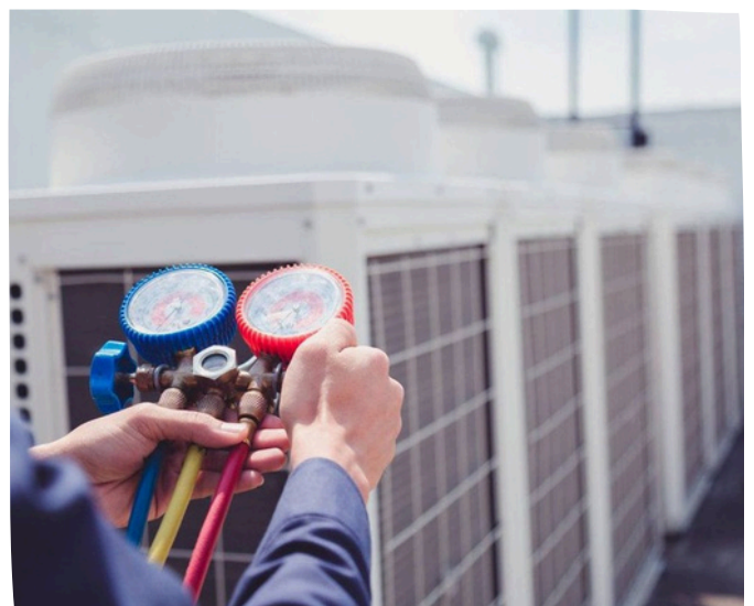
REFRIGERATION SYSTEM INSTALLATION & MAINTENANCE
